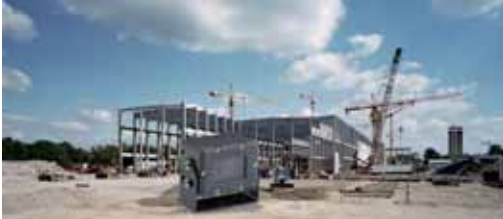
Construction machinery and cranes
